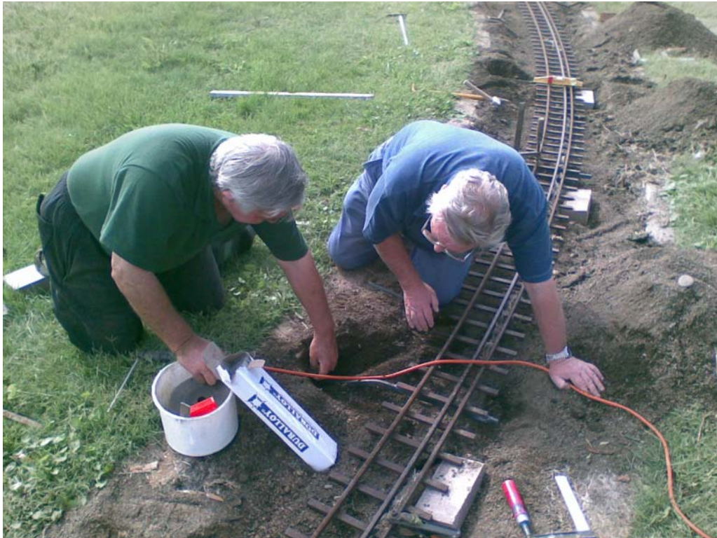
PETER AND BOB WELD EXTENSIONS UNDER THE RAILS TO ASSIST IN MAINTAINING THE CORRECT CAMBER AND ALIGNMENT INTO AND AROUND THE CORNER
