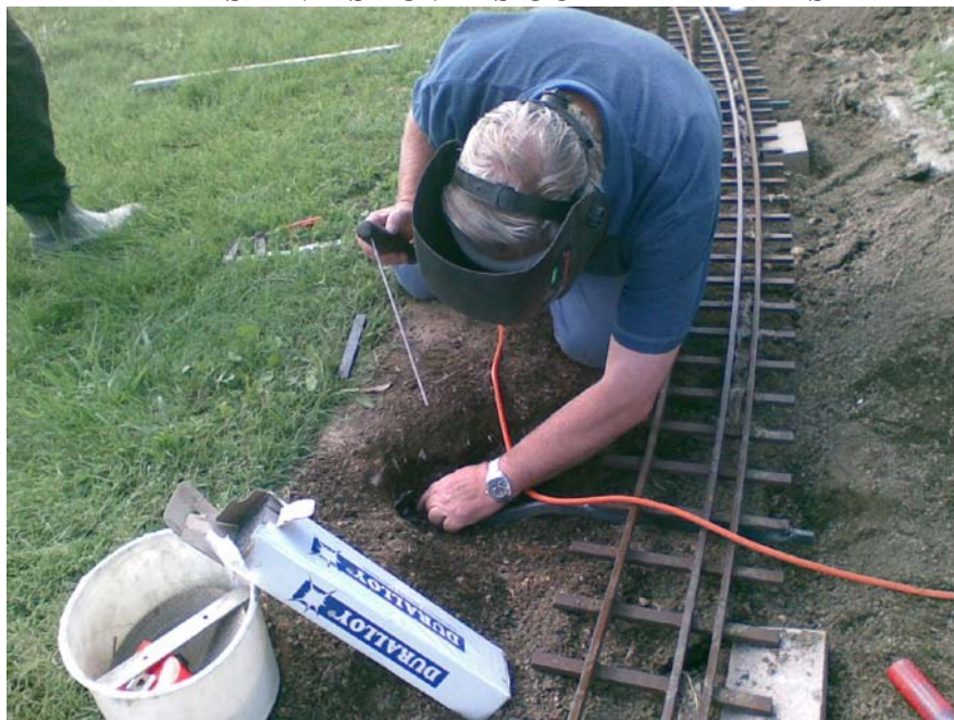
BOB WELDS THE EXTENSIONS ONTO THE TRACK
