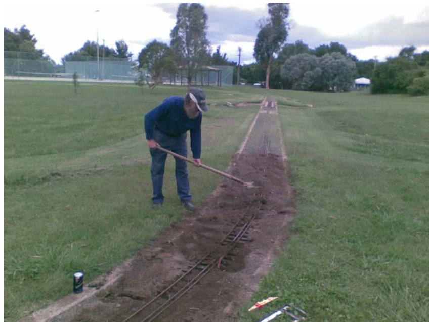
FRED SHOVELS THE BALLAST BACK AFTER THE JOB IS COMPLETE.
